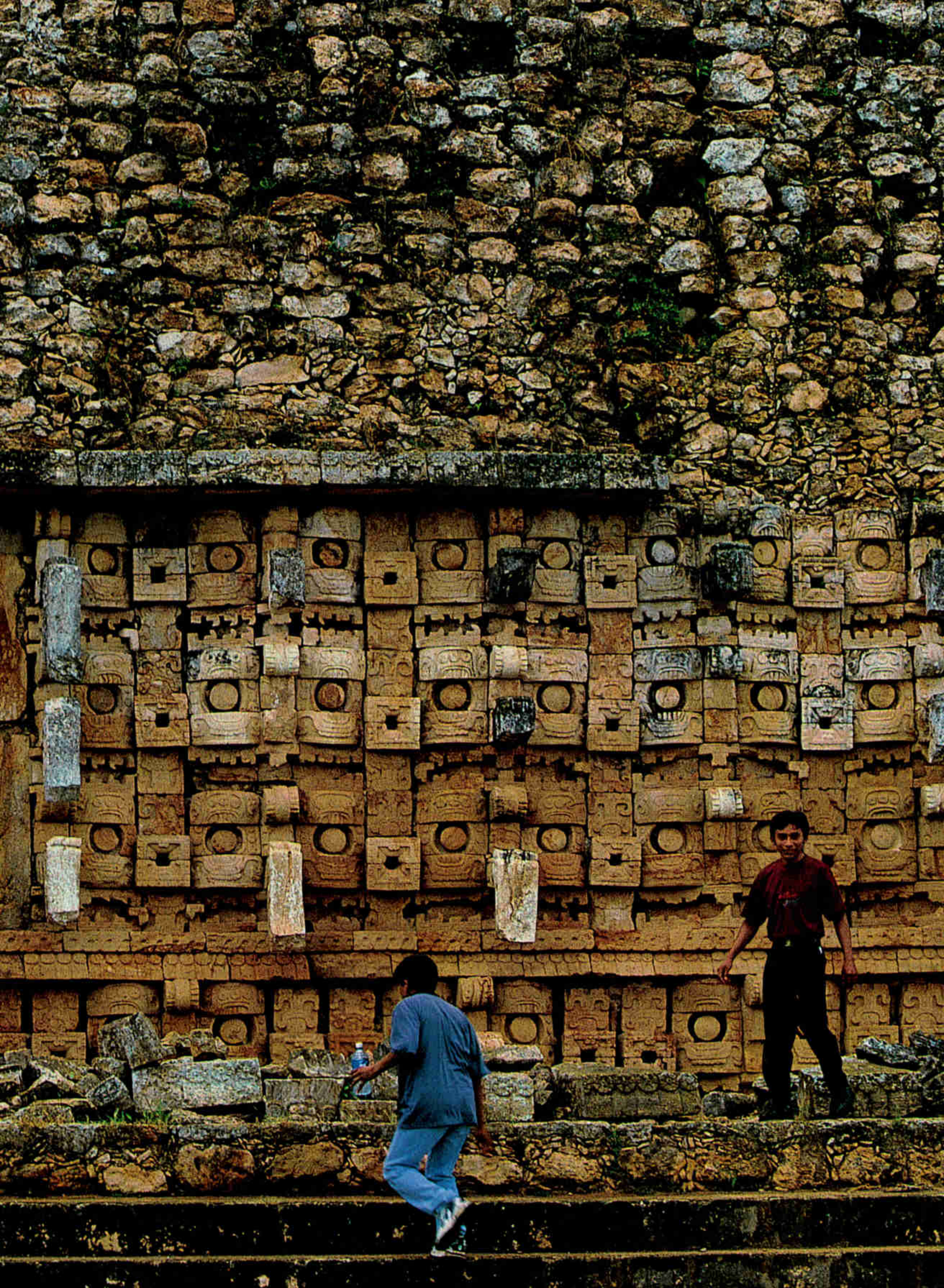
one of the principal buildings at the ruins of Kabah. The cobbled mask-free area, at top, reveals the building's core of mortar and stone that characterizes Puuc architecture.
